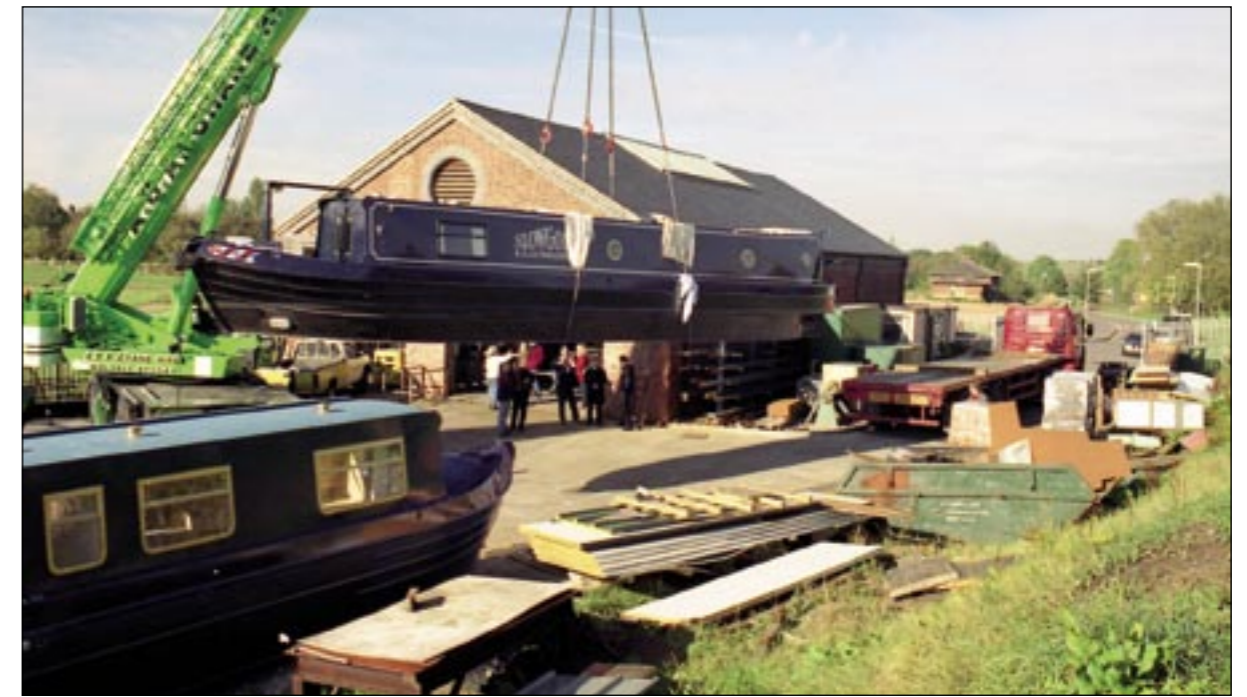
Boatbuilding at Measham
