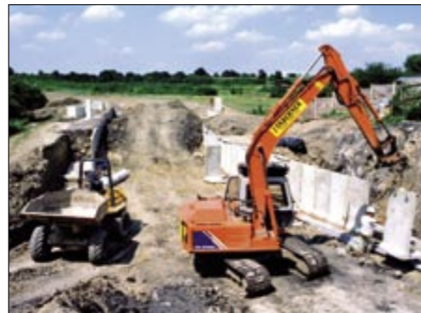
Canal construction at Donisthorpe
